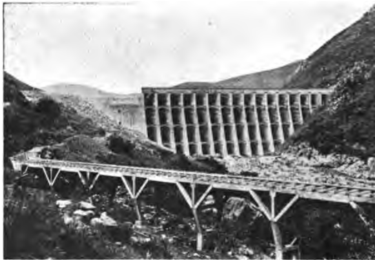
LAKE HODGES DAM FROM BELOW Height 156 feet from bedrock; 750 feet in length.
